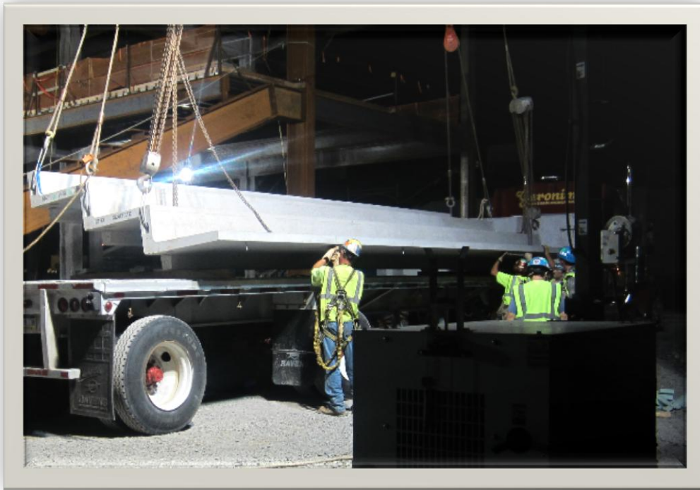
Photo 1: Precast Stadia | Courtesy of Mortenson
